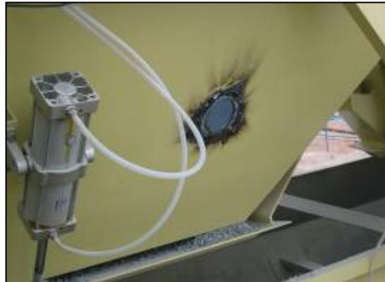
1 Cut the hole
